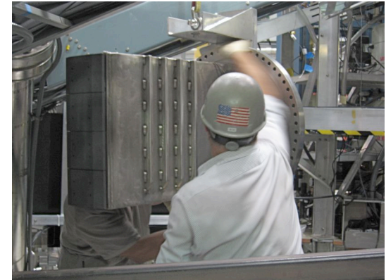
Inconel port cavity with graphite tiles
